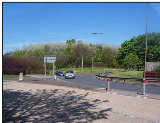
Photograph 4.1 Bugtlin Roundabout southern and eastern approach arms
